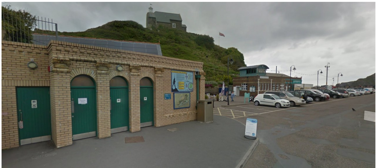
Photo of toilet block (accessible toilet is the first door on the left)
